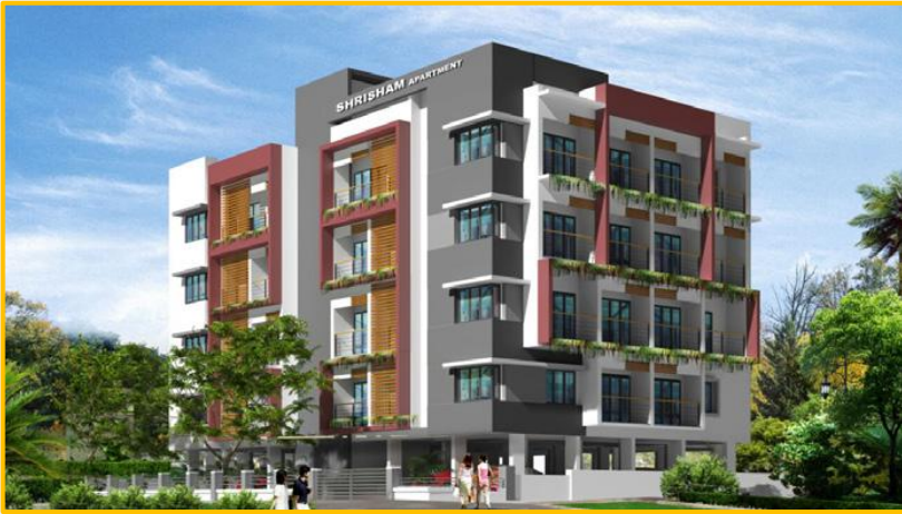
Shrisham Apartment Location: Udupi Client: Aarbee Developers
